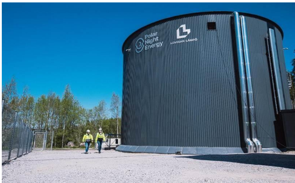
Foto: smilšu akumulators. Avots: TechCrunch ( https://techcrunch.com/2025/06/16/finland-warms-up-the-worlds-largest-sand-battery-and-the-economics-look-appealing )
